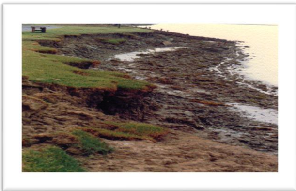
Eroded bank of Nayachara Island
