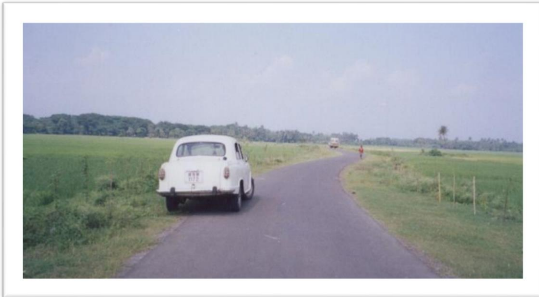
Condition of JGT treated road after 18 months
