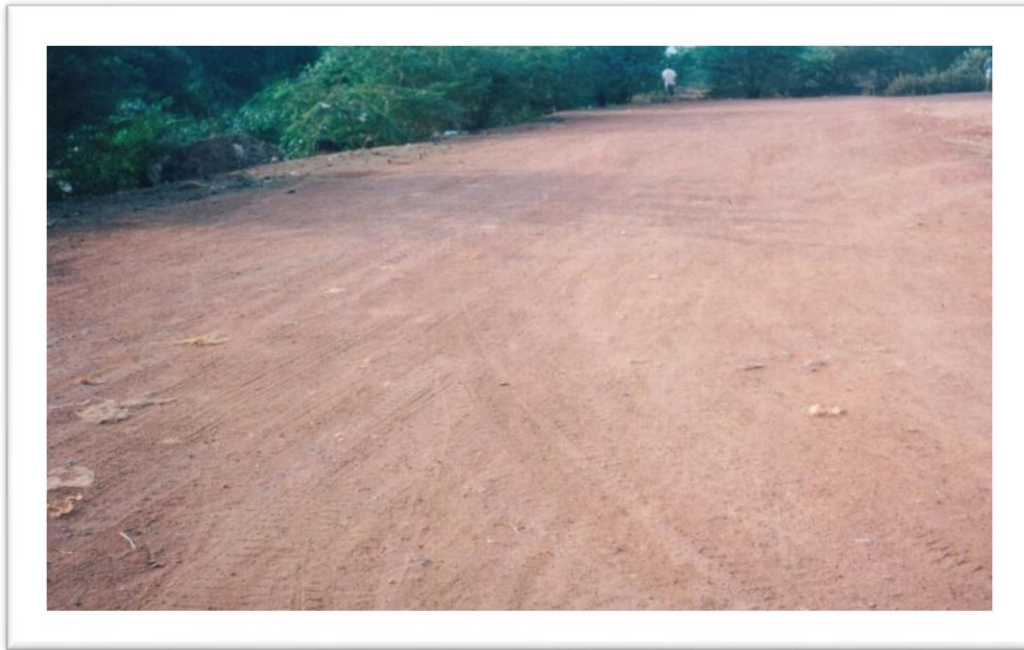
Finished Road after 7 years of construction
