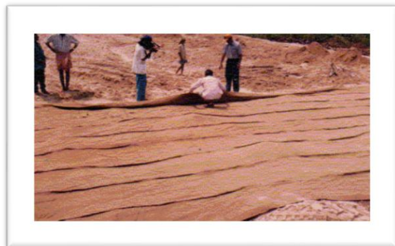
Laying of Jute Geotextile
