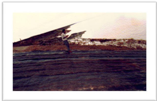
JGT was laid on eroded bank of Nayachara Island
