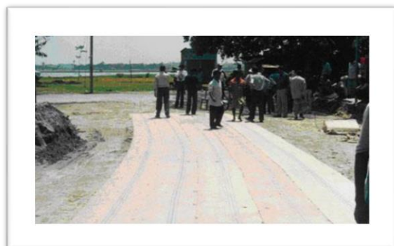
Laying of JGT on road
