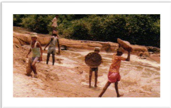
Leveling in progress
