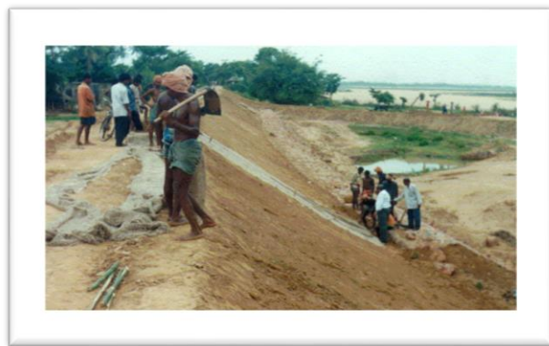
Dressing of Slope & Laying of JGT
