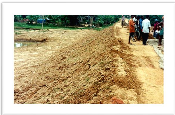
River Embankment at Beluakhali, Bhubaneswar
